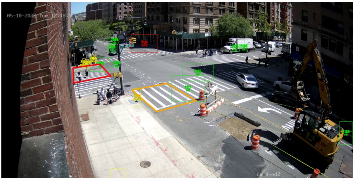
Figure 13 Construction at the Intersection
